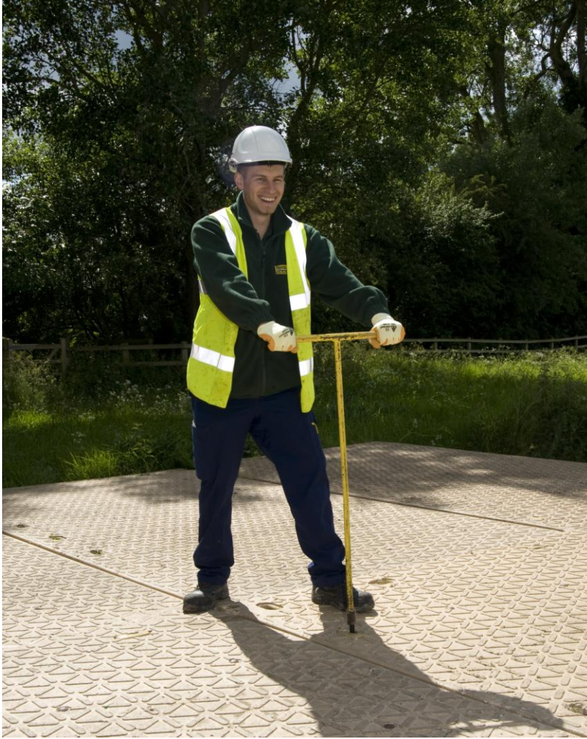
Fig 8 Use T bar to turn pin to lock
