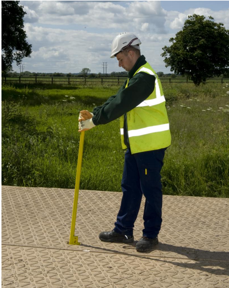
Fig 6 Use pry bar to centre hole
