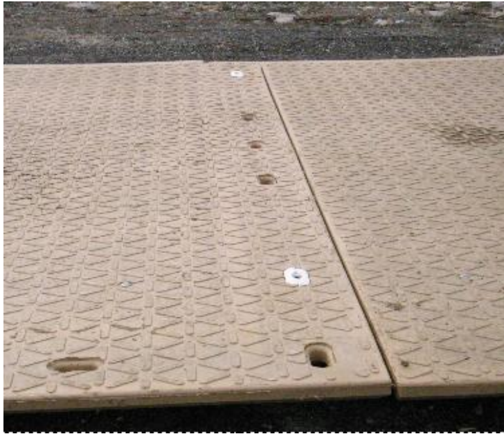
Fig 10 Mat correctly lined up and pinned
