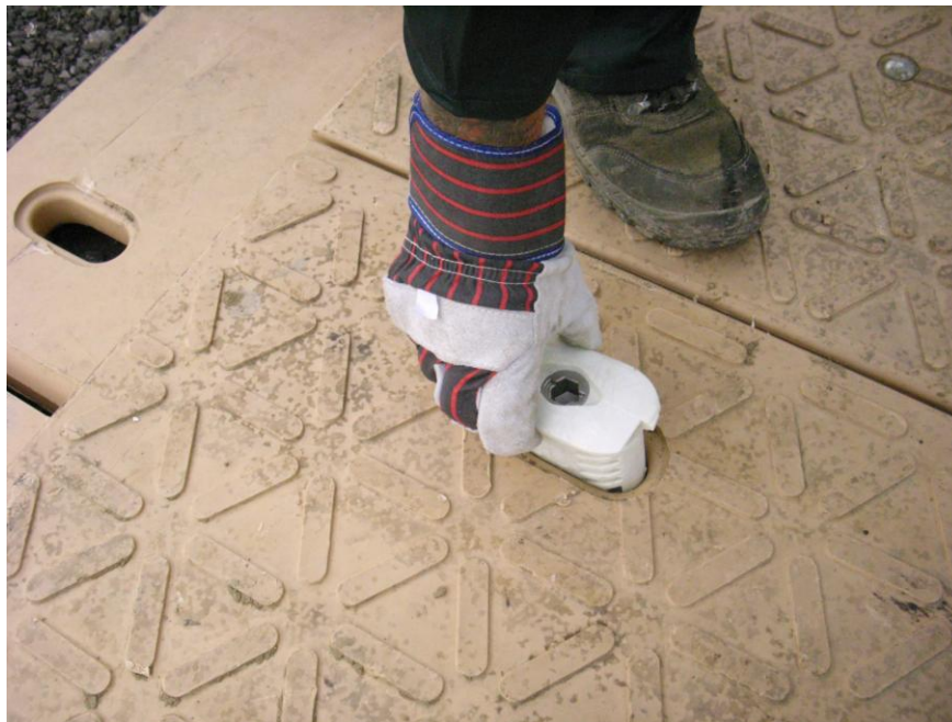
Fig 7 Place pin in pin hole
